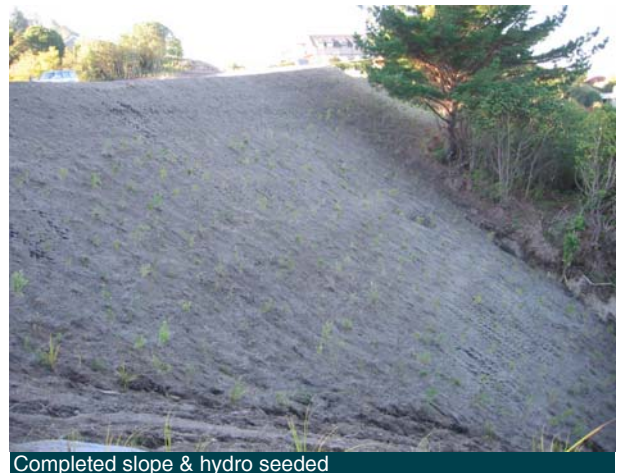
Completed slope & hydro seeded
