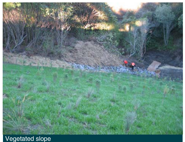
Completed slope & hydro seeded
