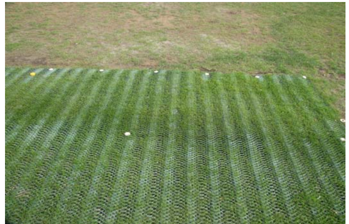
Grass Protecta laid over prepared surface
