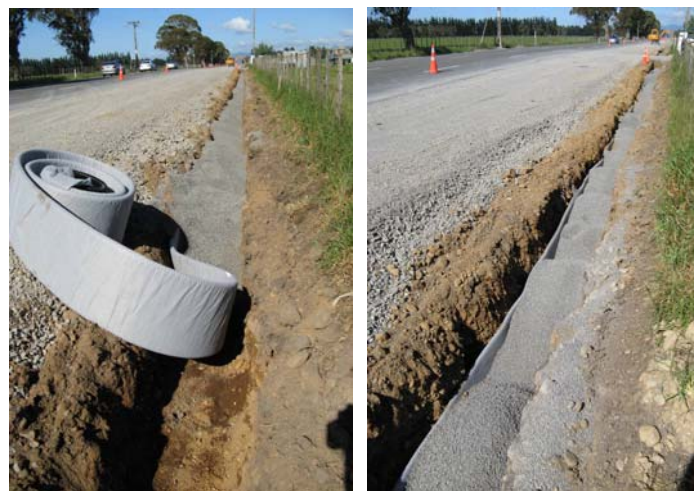
Laying of Megaflo on the edge of the trench
