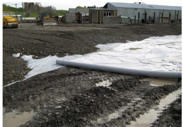
Laying bidim and river run
