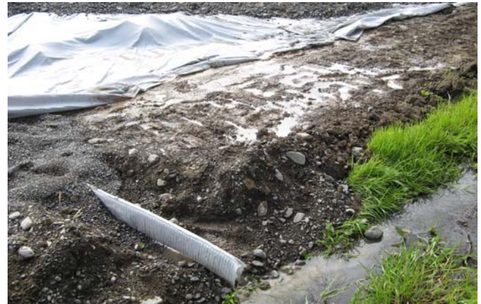
Megaflo 150 exit into drain
