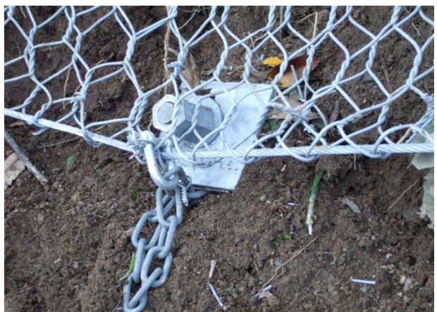
Anchor at the toe of the slope
