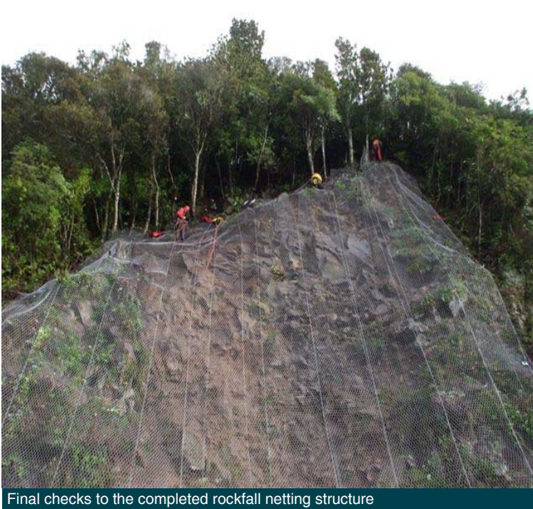
Completed rockfall netting structure
