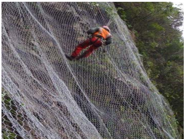
Avalon staff abseiling down the slope to place anchors
