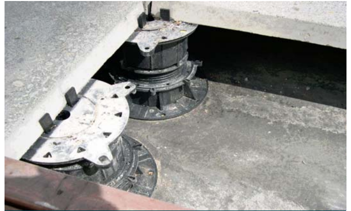
VersiJacks on waterproofing membrane
