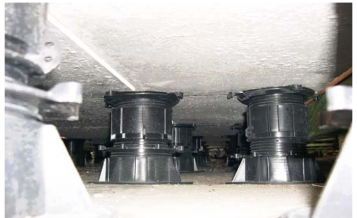
VersiJacks supporting pavers (underside)
