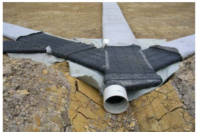
Installing Megaflo® with Dual Herringbone Fittings
