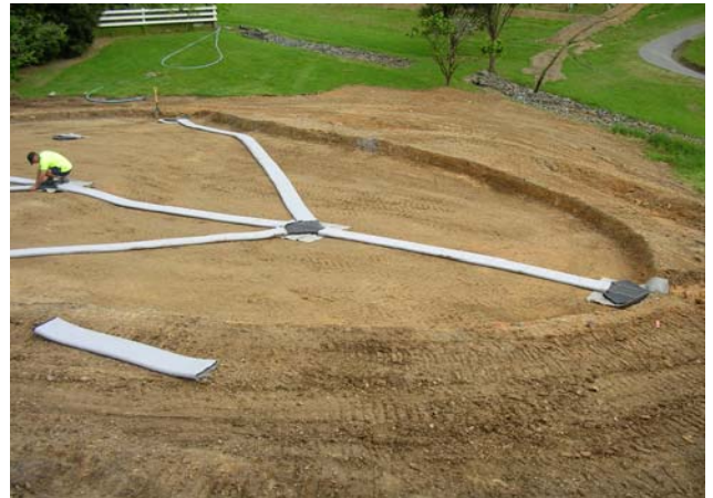
Placing Megaflo® onto the prepared profile
