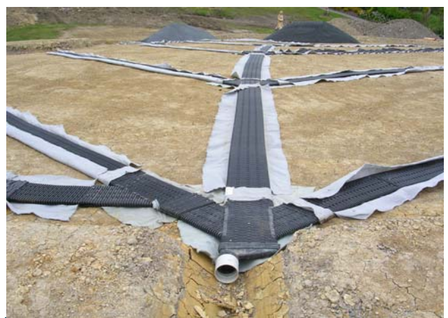
Megaflo® 300 with bidim® geotextile sliced open
