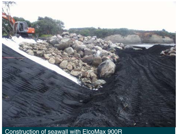
Construction of seawall with ElcoMax 900R
