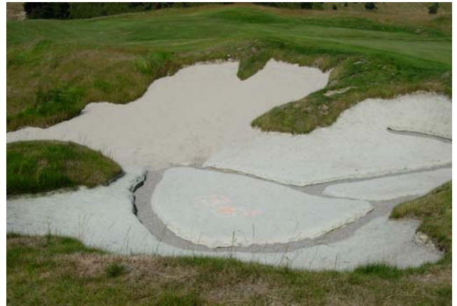
Laying of BunkerMat and Sand
