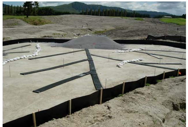
Laying of Megaflo
