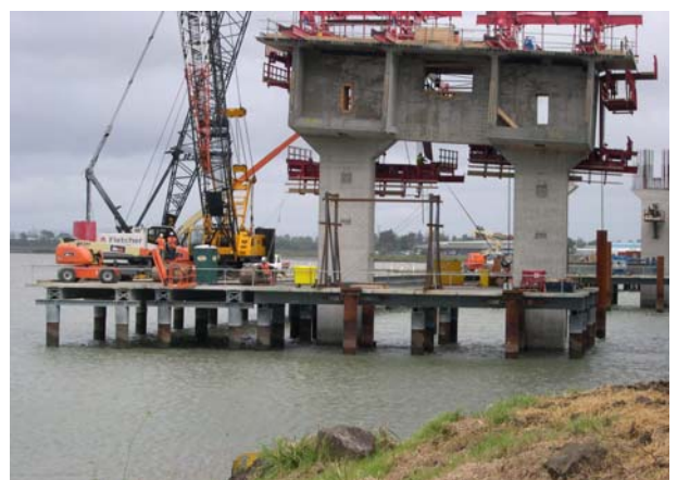
Temporary platform landing constructed
