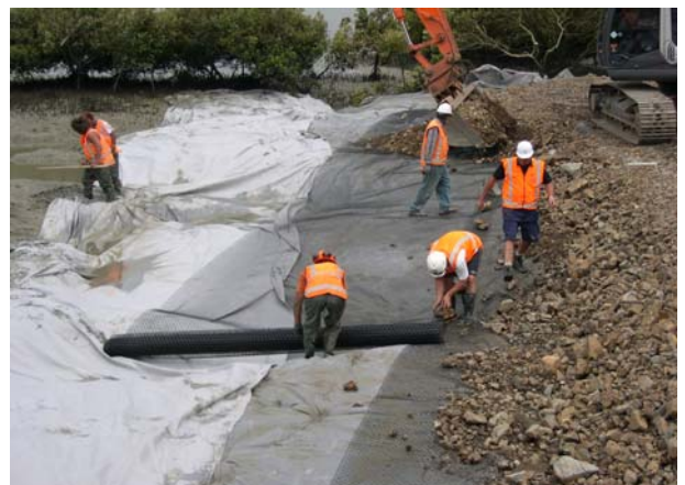
Placement of Tensar TriAx and bidim for landing
