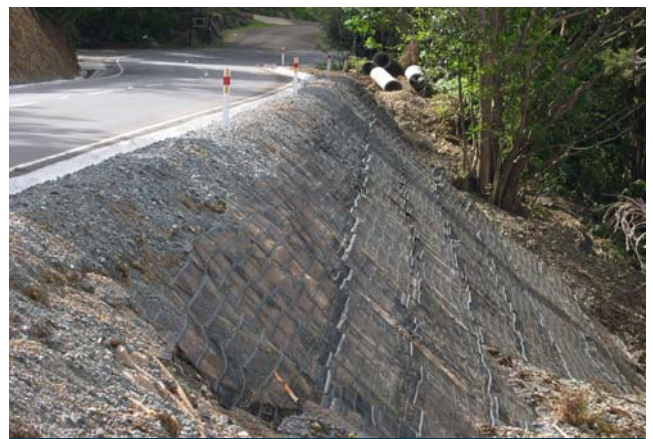
Laying Bidim, Biomac and Tensar
