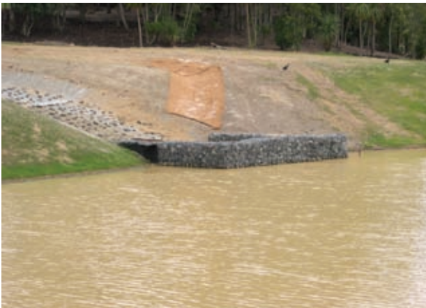
Gabion outlet structure at sediment pond Date: Mar 2008
