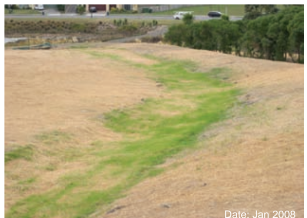
Enkamat & Biomac lined spillway with grass now striking Date: Jan 2008
