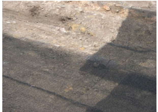
Enkamat placement in spillway subgrade Date: Jan 2008
