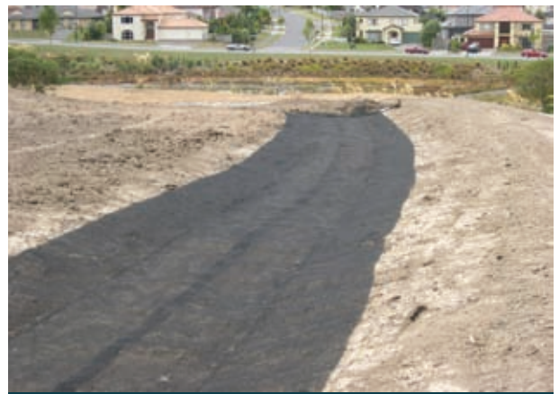
Finished placement of Enkamat Date: Jan 2008
