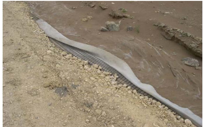
Tensar geogrid for subbase stabilisation
