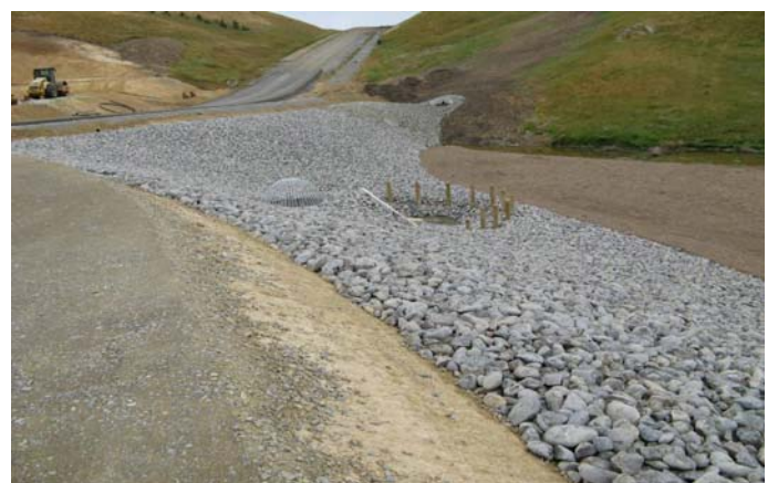
Bidim geotextile under rock rip rap
