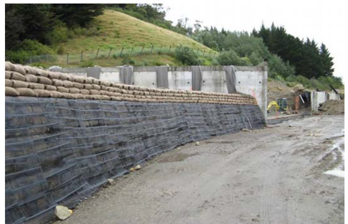
Wrapped slope with hessian bags
