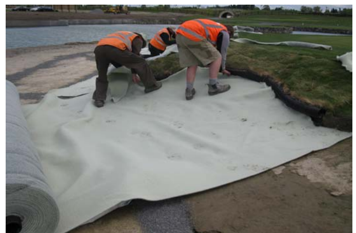
Installing BunkerMat
