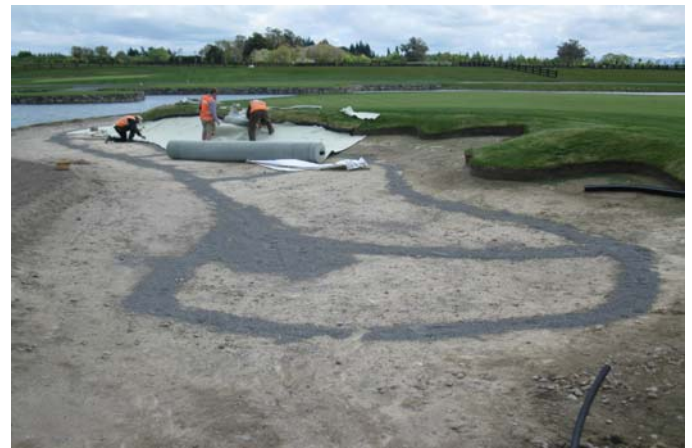
Preparing the bunker
