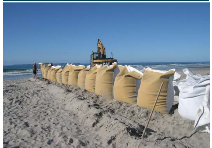
ELCOROCK filled for sewing closure and placement
