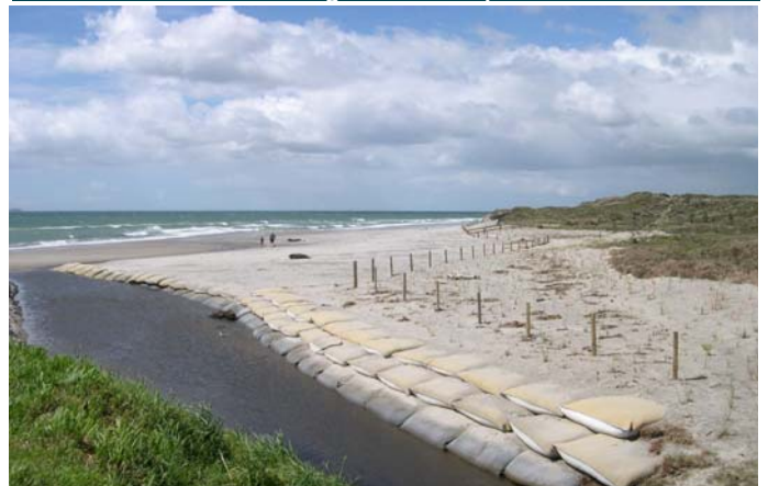
Completed with dune planting and fencing
