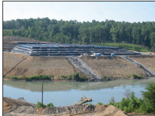
Each bag field accommodated four levels of stacked Geotube® units. The project was designed so that the bags on the bottom level were systematically filled from one side to the other, allowing the second level bags to be placed safely on top of the bottom layer. This continued until the fourth layer was added (above right.)
