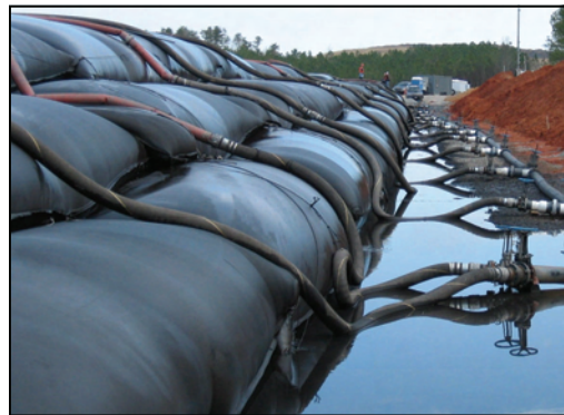
This multiple manifold system controlled the flow of slurry between the Geotube® units.
