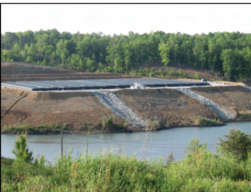
Each bag field accommodated four levels of stacked Geotube® units. The project was designed so that the bags on the bottom level were systematically filled from one side to the other, allowing the second level bags to be placed safely on top of the bottom layer. This continued until the fourth layer was added (above right.)
