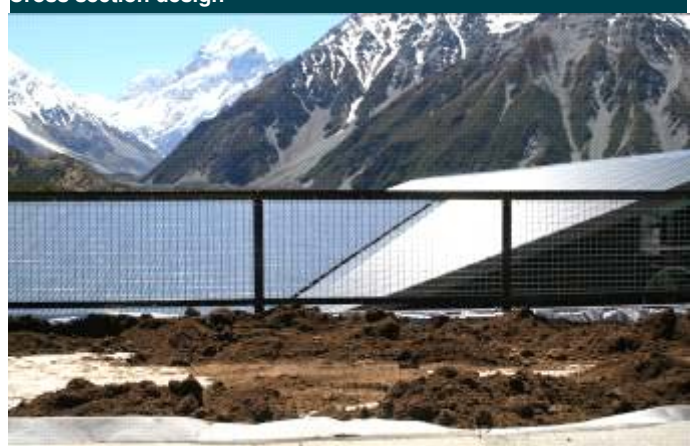
Placement of soil for grass area
