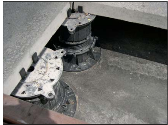
VersiJacks supporting pavers (underside)
