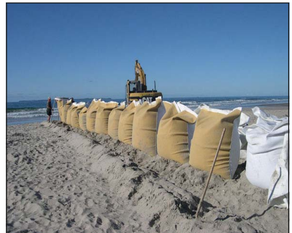
ELCOROCK filled for sewing closure and placement
