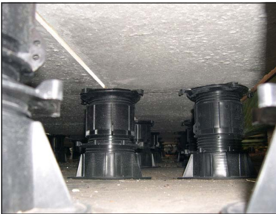
VersiJack on waterproofing membrane
