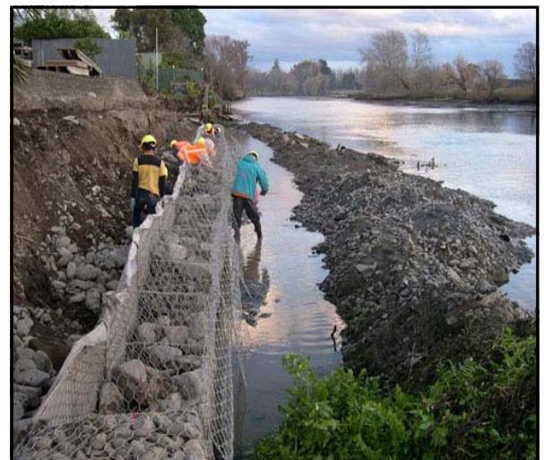
Gabion installation in process
