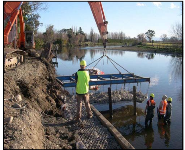
Installation of Reno mattresses
