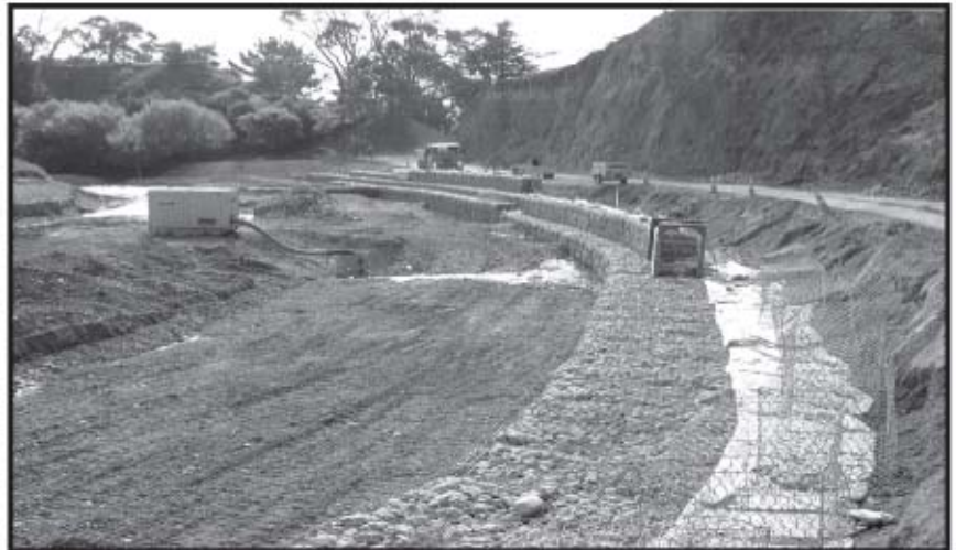
Gabion and Reno Mattresses under construction
