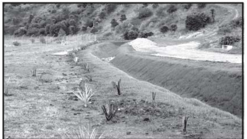
Revegetation of newly completed Enkamat spillway channel
