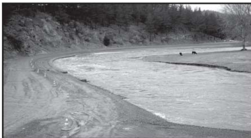
Final works in flood
