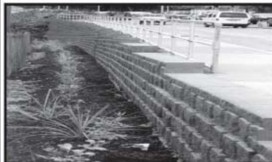
Completed Segmental Retaining Wall
