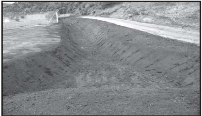
Seed and topsoil placed in Enkamat
