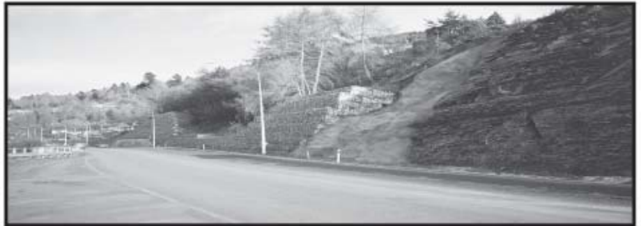
SH6A with the Completed Gabion Walls
