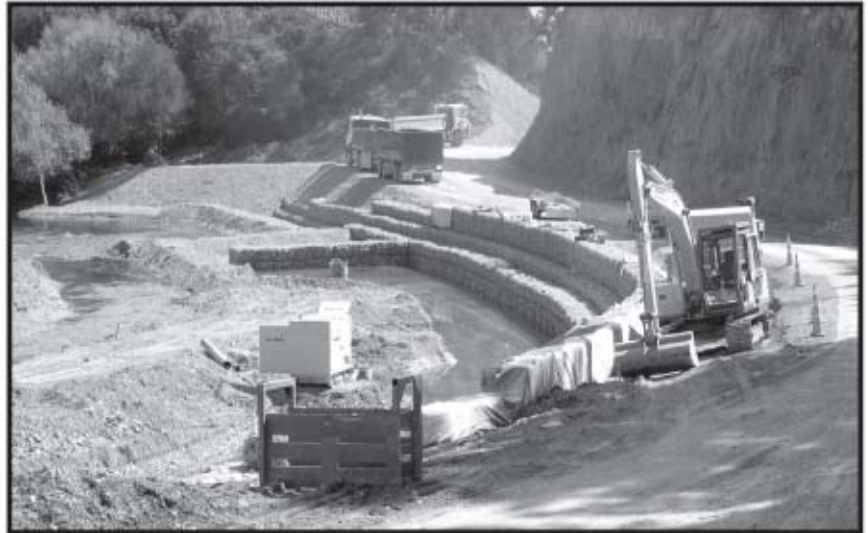
Gabion and Reno Mattresses under construction
