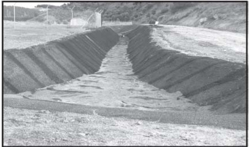
Enkamat secured prior to seed and topsoil placement
