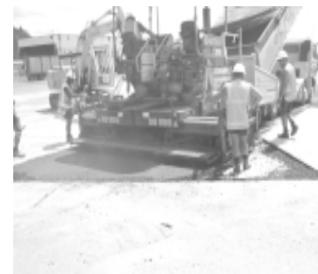
Laying of Asphalt over Tensar ARG
