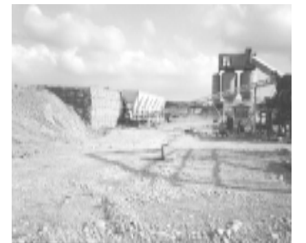
Pond Road Batching Plant for Fulton Hogan - Christchurch
