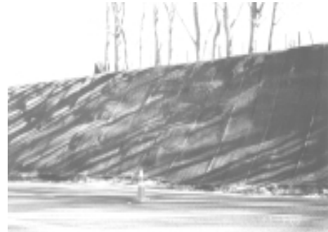
Enkamat and Rockfall Netting in place
