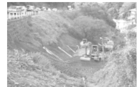
Site view during construction
