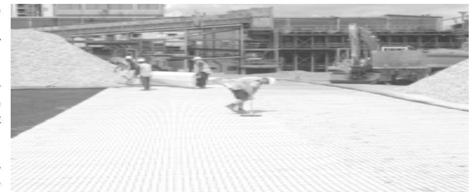
Tensar ARG being placed prior to A.C. overlay
