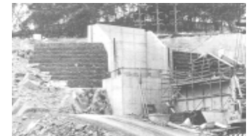
Terramesh Wing Walls - Hall Quarry - Boral Resources, Canberra
