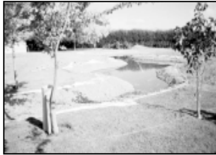
Bentofix with gravel cover prior to filling
