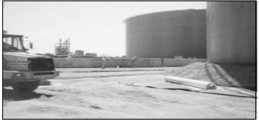
Placement of Bentofix over HDPE liner
