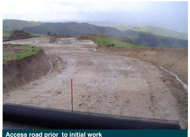
Access road prior to initial work
