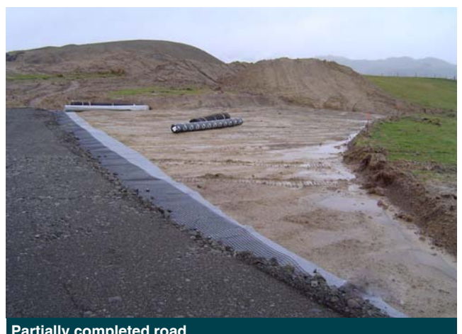
Partially completed road
