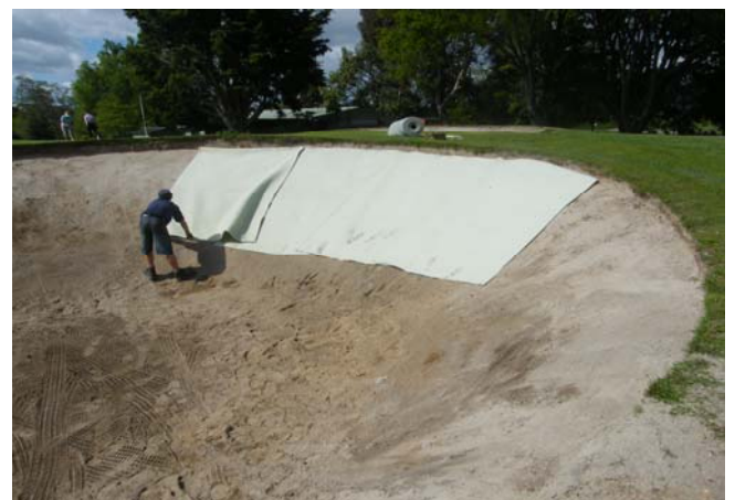
Installing BunkerMat
