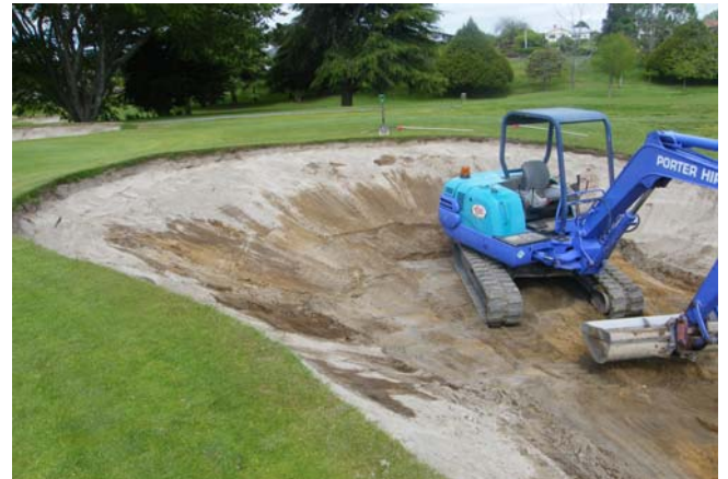
Preparing the bunker
