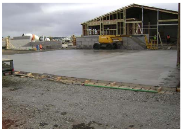
Completed SFRC Floor Slab
