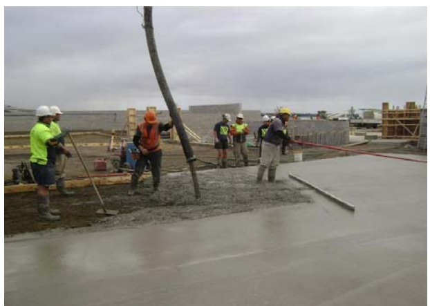
Pouring of concrete
