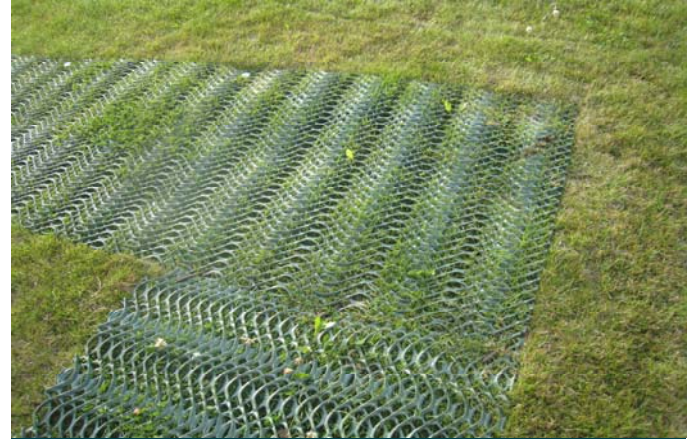
GrassProtecta laid directly over turf
