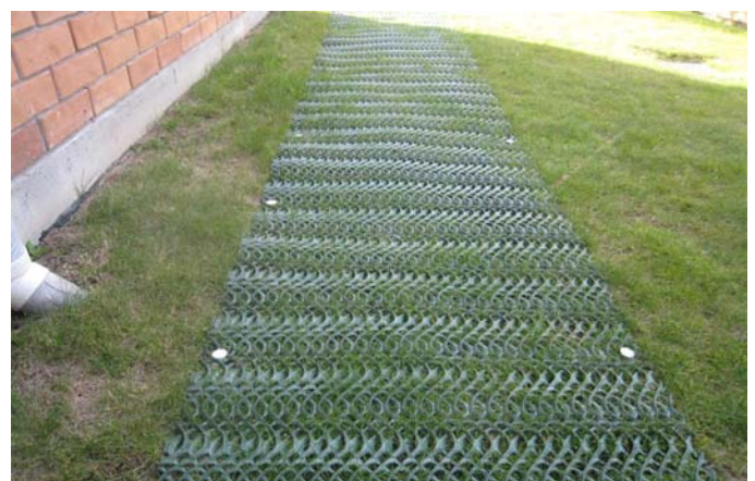
GrassProtecta secured to the ground with 175mm BioPegs
