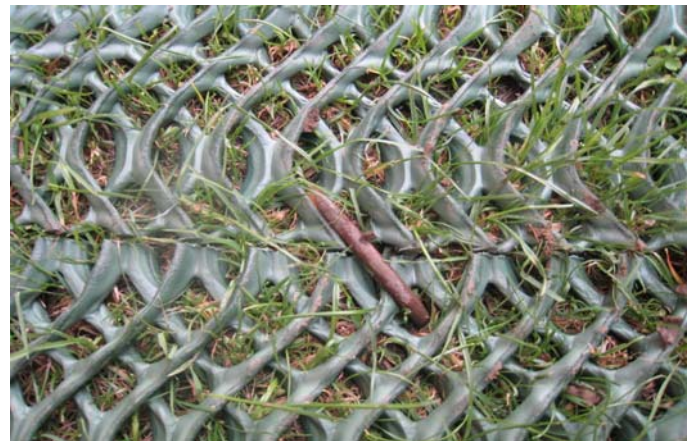
GrassProtecta secured to the ground with 170mm "U" pins
