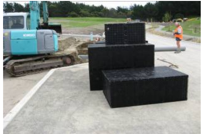
Initial site with VersiTanks
