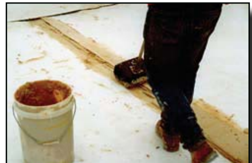
Applying the bentonite Fillet
