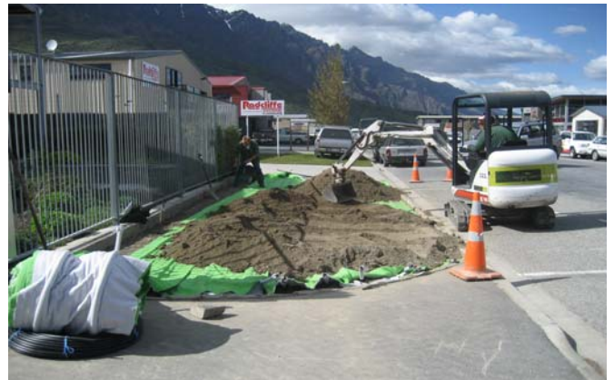
Placement of ECO Rain® and topsoil
