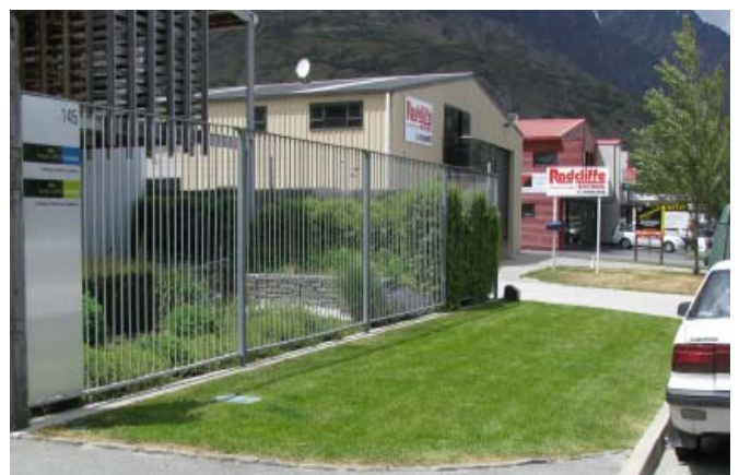
Completed grass frontage area
