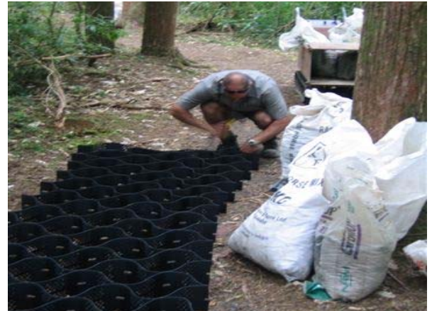
Expansion of Geoweb sections
