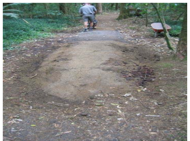
Geoweb melds with the undisturbed track
