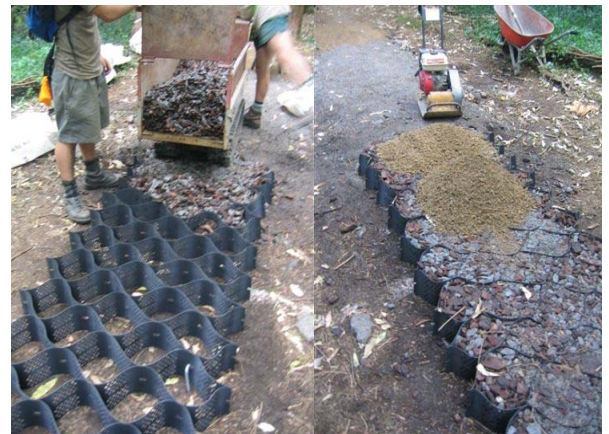
Placement of combination of GAP50 and bark
