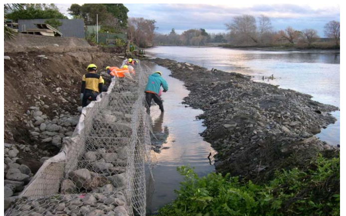
Gabion installation in process
