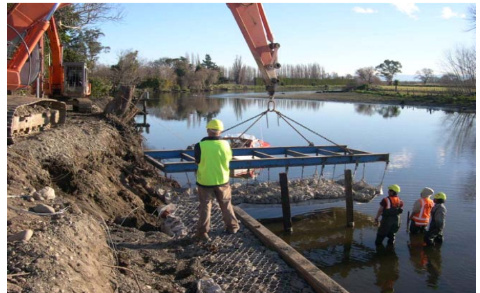
Installation of Reno mattresses
