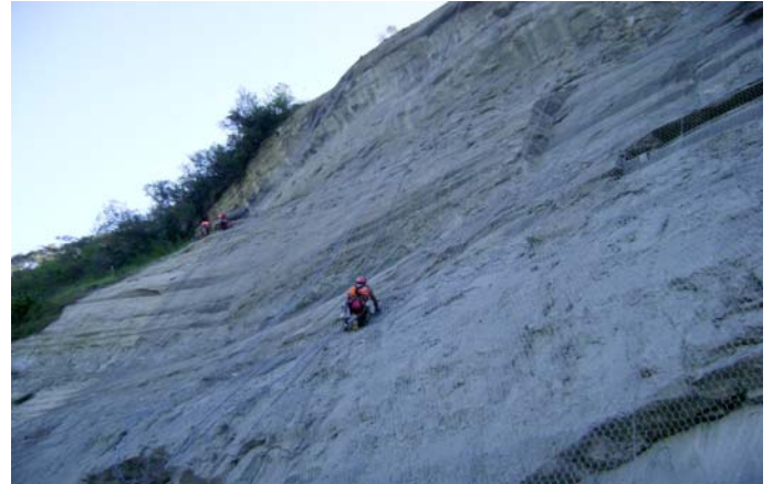
Avalon abseilers installing rockfall netting
