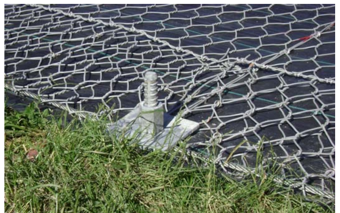
Anchors at the top of the slope to hold the netting
