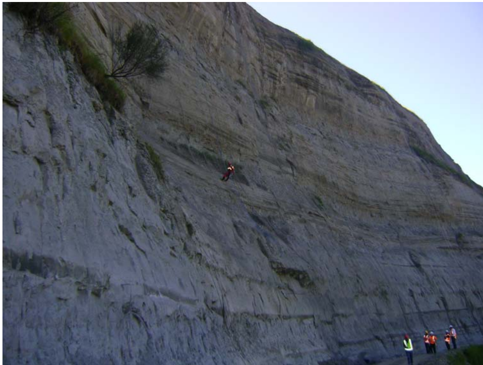
Rockfall netting installation by Avalon abseilers near completion
