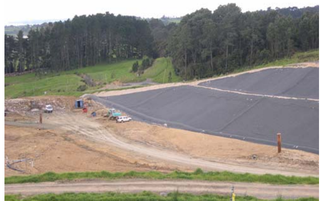
Whitford Landfill in use
