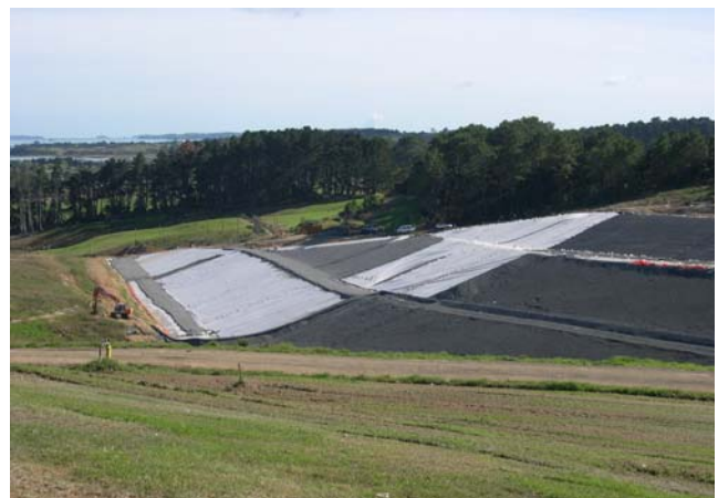
Laying of HDPE, Polyfelt and ElcoSeal
