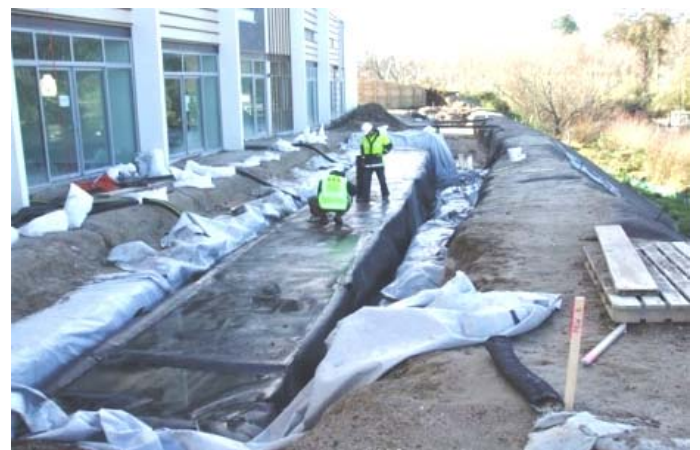
Waterproofing of VersiTanks with HDPE liner Date: June 2008
