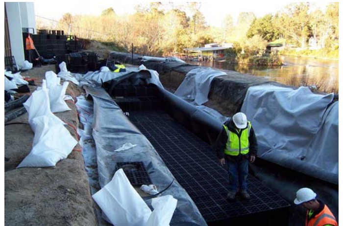
Placement of VersiTanks along the Waikato river Date: June 2008
