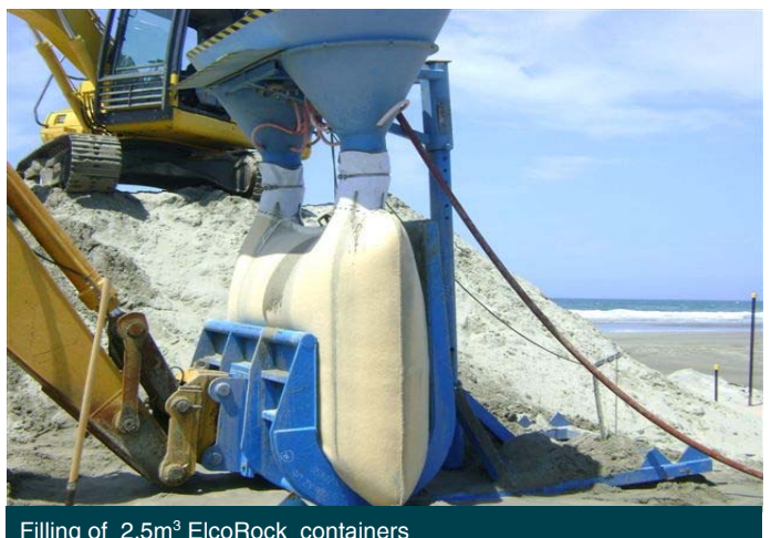
Filling of 2.5m 3 ElcoRock containers
