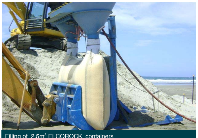
Filling of 2.5m 3 ELCOROCK containers
