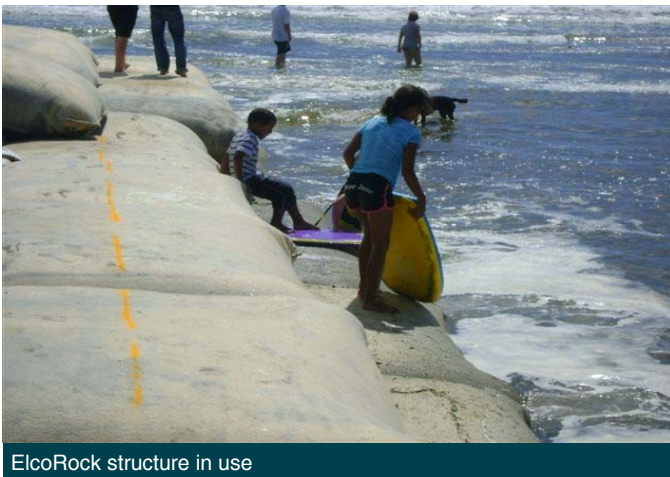
Final ElcoRock wall structure
