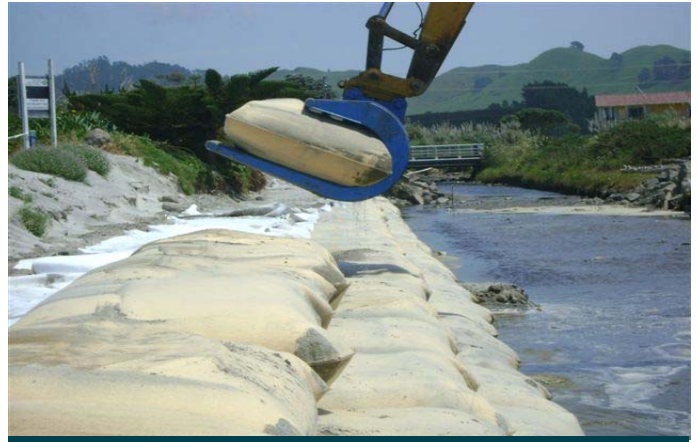
Placing of ElcoRock containers
