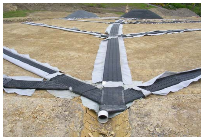
Megaflo® 300 with bidim® geotextile sliced open
