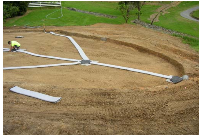
Placing Megaflo® onto the prepared profile
