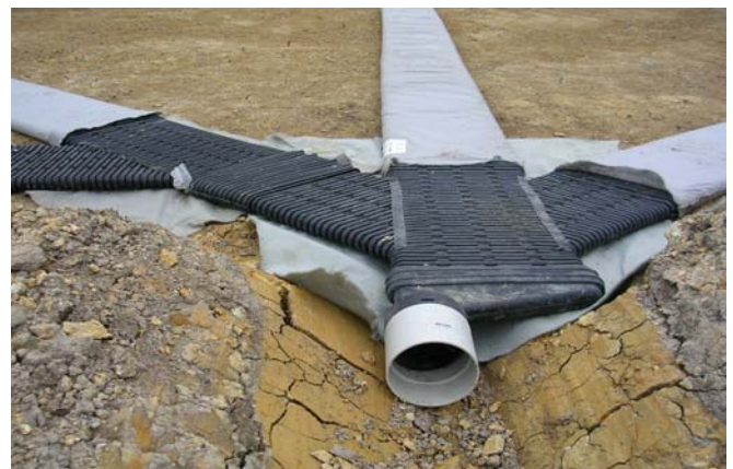
Installing Megaflo® with Dual Herringbone Fittings
