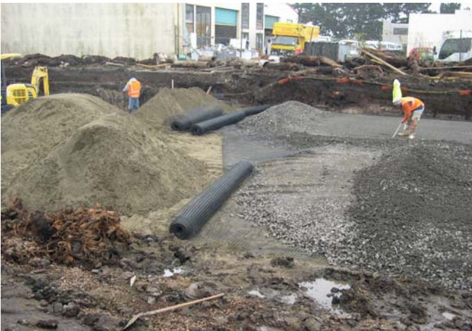
Laying of Tensar geogrid
