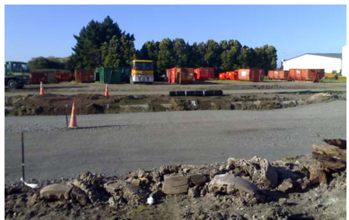
Placement of GAP 65 sub-base course
