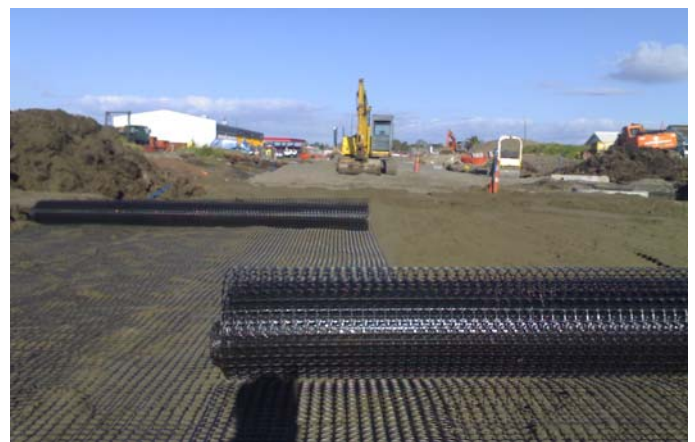
Laying Tensar geogrid
