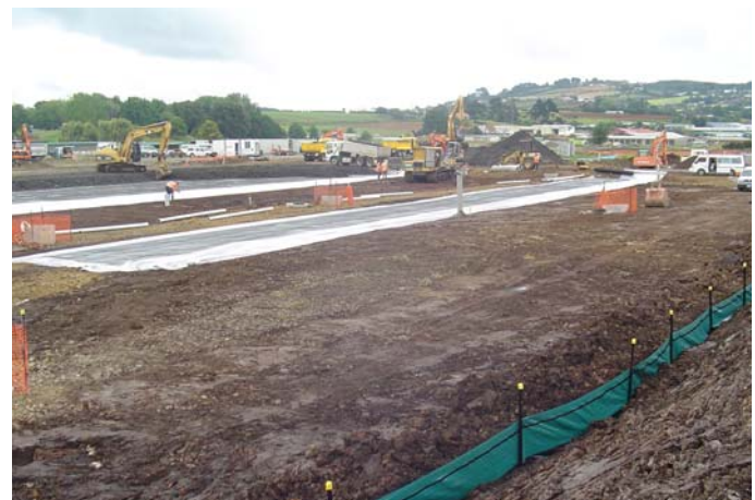
Bidim and Tensar placement
