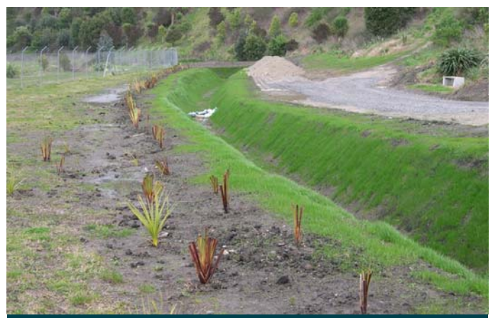
Revegetation of Enkamat lined slopes
