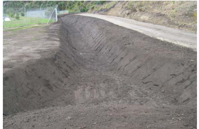
Channel prior to construction
