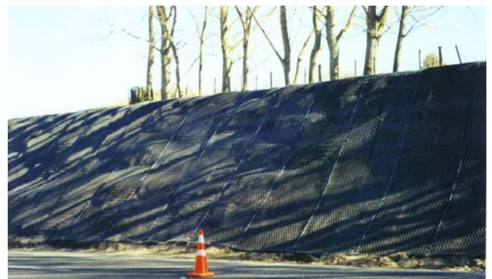
Enkamat and Rockfall netting in place
