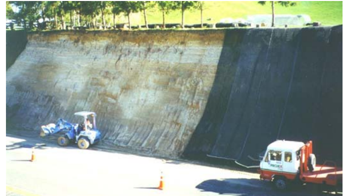
Placement of Enkamat
