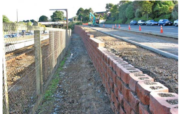
Wall during construction
