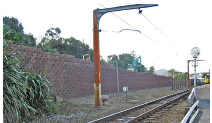
Wall view from station
