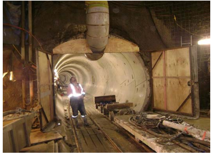
View of Hobson Bay Tunnel from the Shaft
