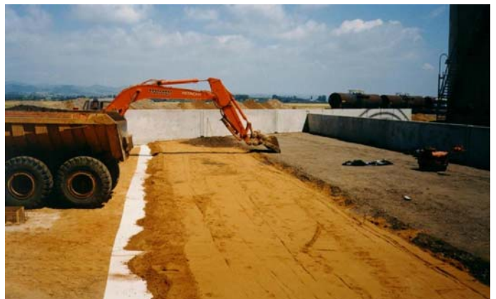
Fill placement over Elcoseal
