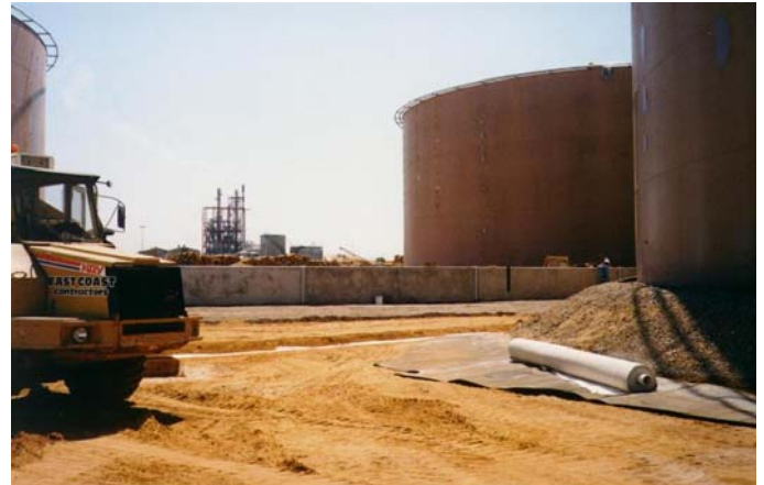
Placement of Elcoseal over HDPE
