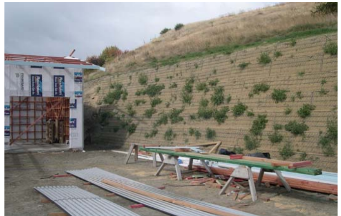
Overall view of Green Terramesh slope
