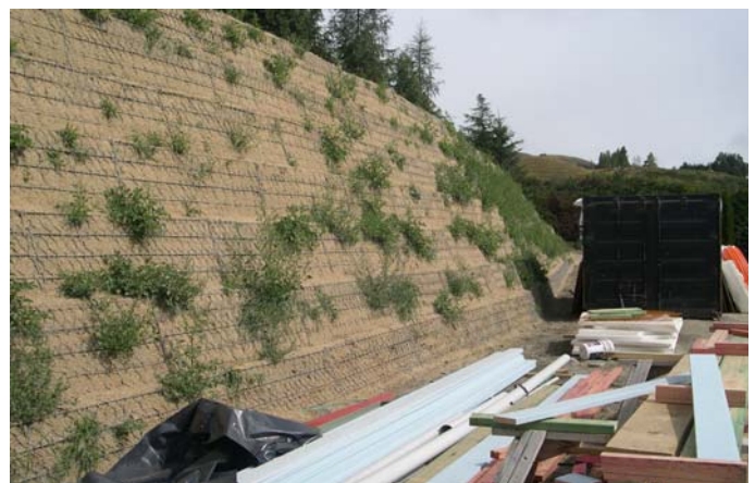
Vegetation starting to grow prior to hydroseeding
