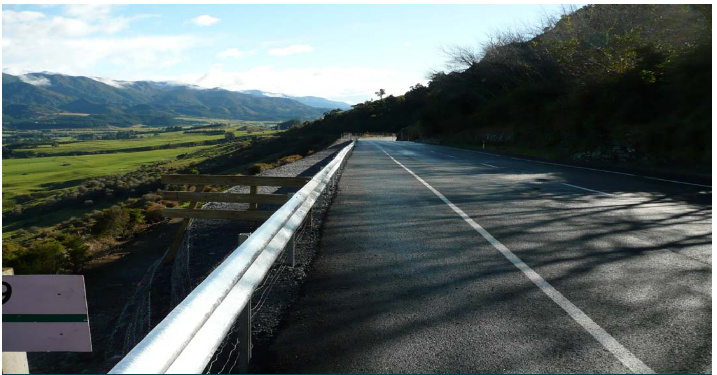
Completed project and road reopened
