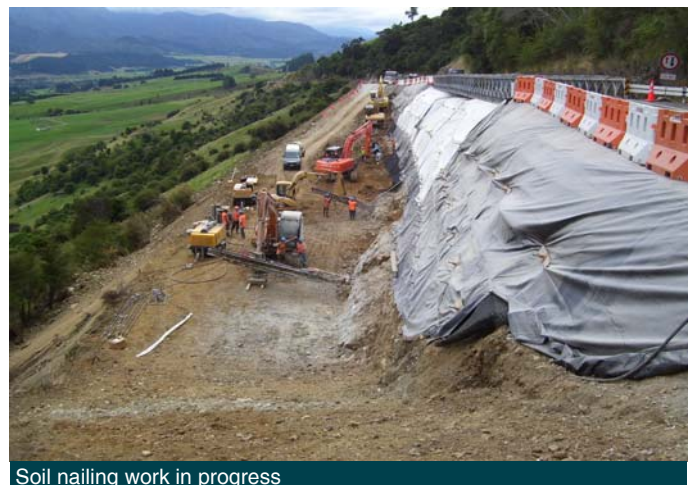
Soil nailing work in progress
