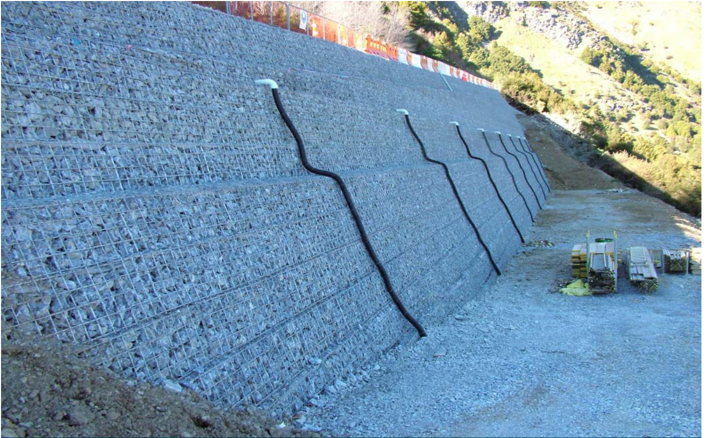
Completed Green Terramesh structure
