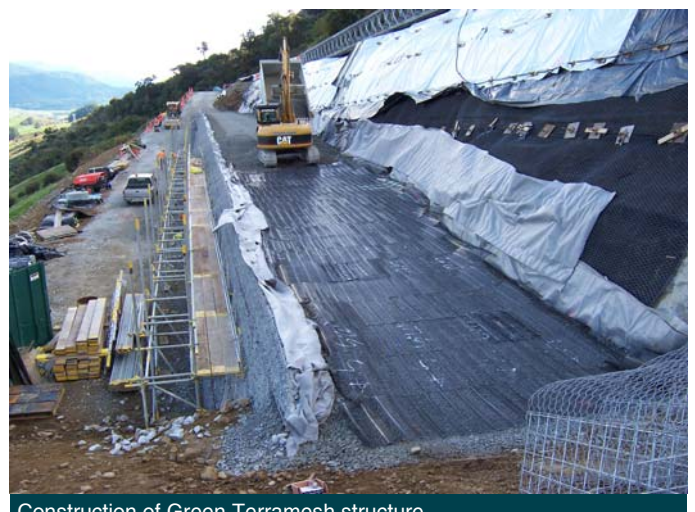
Construction of Green Terramesh structure
