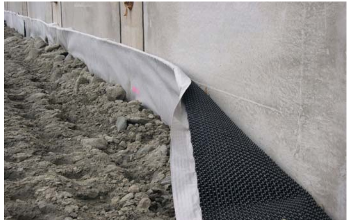
Installation of Cordrain against the concrete wall
