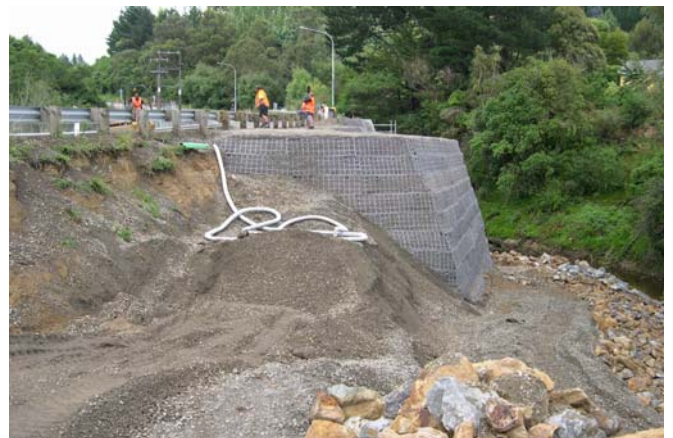
Construction of Green Terramesh Structure
