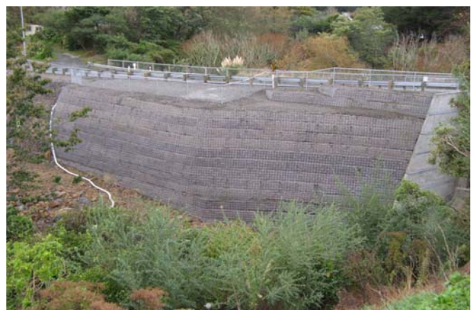
Completed Green Terramesh Structure at Bryants Bridge
