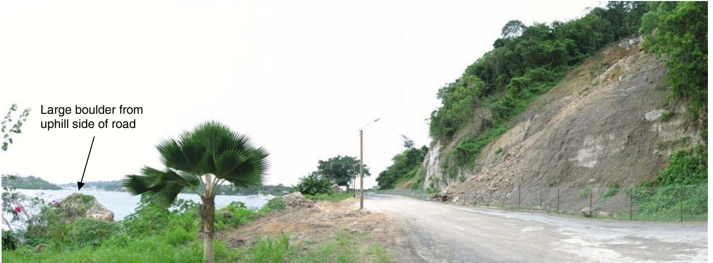
Landslip along Wharf road
