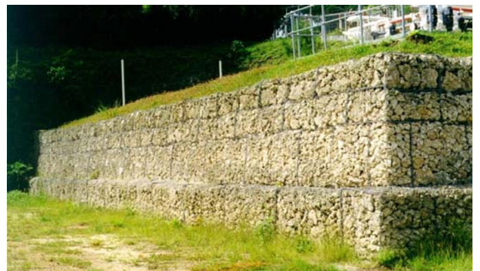
Gabion Wall after construction
