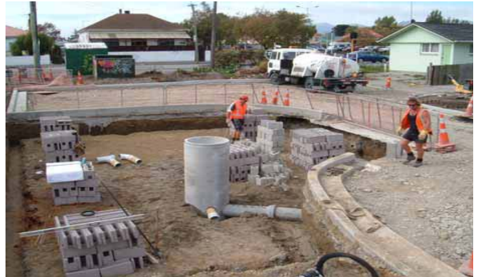
Construction of rain garden
