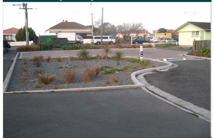
Rain garden completed / in use
