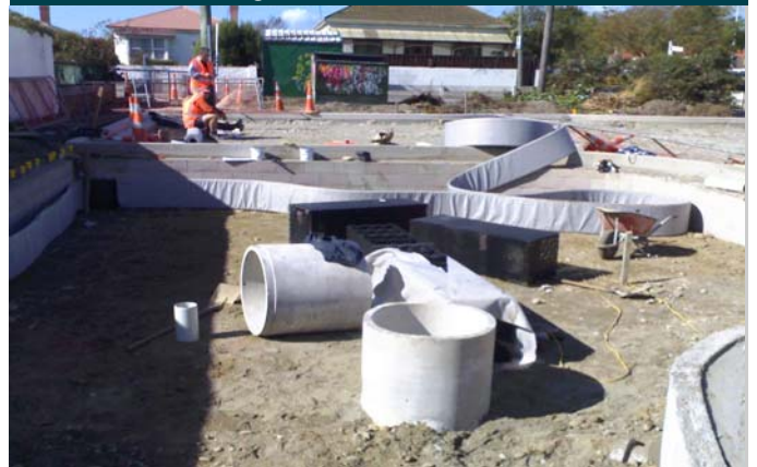
VersiTanks & Megaflo being fitted
